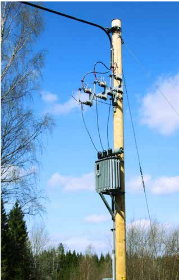
Pole-mounted substation.
