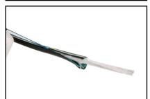
Ring cut the tube with a tool which is intended for the purpose. Applying wrong tools can damage the fibers. The length to be opened in this operation is determined by the splice box that you intend to use.
