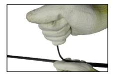
Measure and mark the length of the cable to be opened up. The length is determined by the splice box that you intend to install the cable in. See installation instructions for the box you have chosen. For example 1.5 m, when using Nexans splice box NS2.
